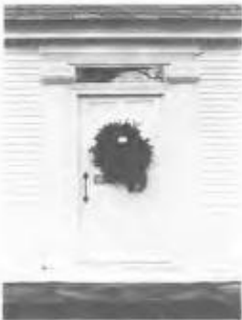
This elaborately detailed Cape Cod type house (49) was built in 1793 for Daniel Hulett, who fought in the Revolution at the Battle of Saratoga. The central paneled door is framed by an unusual Federal style surround, and running under the eaves is an intricate denticulated cornice.
