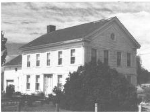
Described in 1867 as "elegant and commodious," this house (6) was built a few years earlier for David G. Blossom on his father's farmstead. Once wrapped around by a sweeping Italianate style porch, it remains distinctive for its corner pilasters with round arch panels, handsome front door, and first floor walls sided with flush boards.
