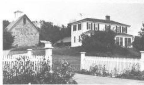
The large, c.1800, Georgian plan house (1) on this property in the northwesternmost corner of Pawlet sharply contrasts with the large barn behind it. Likely built in the 1880s, the barn was covered with slate that may have come from a nearby quarry. The name of the farm, "Mount Pleasant," is spelled out in red slate on the front gable end.
