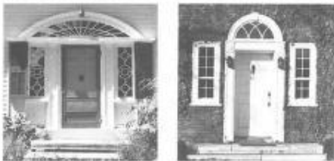
Among the most distinguished Federal style buildings in Pawlet are two, large, hip-roofed houses. Dr. John Sargent's home (57), part of a large farm, was built in wood in 1799, while the Leach family house (55, 1810) is brick. Both are elegantly detailed with Doric friezes under the eaves and two, formal, five-bay wide facades—one with a transom over the central door and one with a fan and sidelights.
