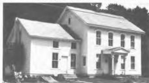
Riddling the landscape of West Pawlet are a number of slate quarries, some more than 175 feet deep. Quarry sheds at this site (4) in the northwest corner of town date from around 1900. One of the most prominent slate quarrying firms was Rising and Nelson, still in operation. Its founding partners were neighbors in West Pawlet. Simeon Rising's wood-frame home (A42, c.1880) is detailed with Italianate style segmental arch windows on the second floor and cornice brackets under the eaves.
