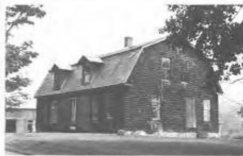
Scattered throughout Pawlet are several early houses built with gambrel roofs. The gambrel form, uncommon in Vermont, may have been brought to the area by settlers from the Hudson River valley where it was used more extensively. This house (40, c.1800) has been slightly altered by the addition of slate roofing and wood shingle siding.
